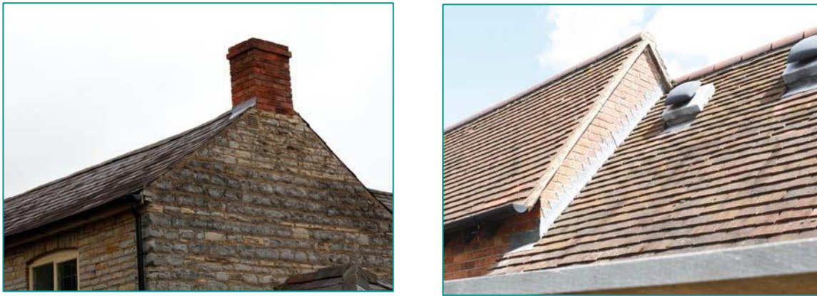
Fig. E14 - Examples of 'wet verge' using mortar to secure the roof tiles.
