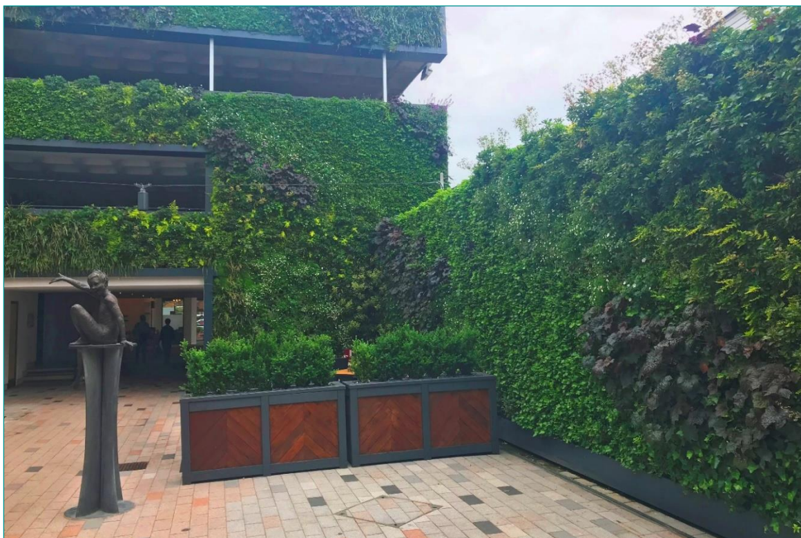
Fig. E26 - Living/Green Wall in Bell Court Stratford-upon-Avon.
