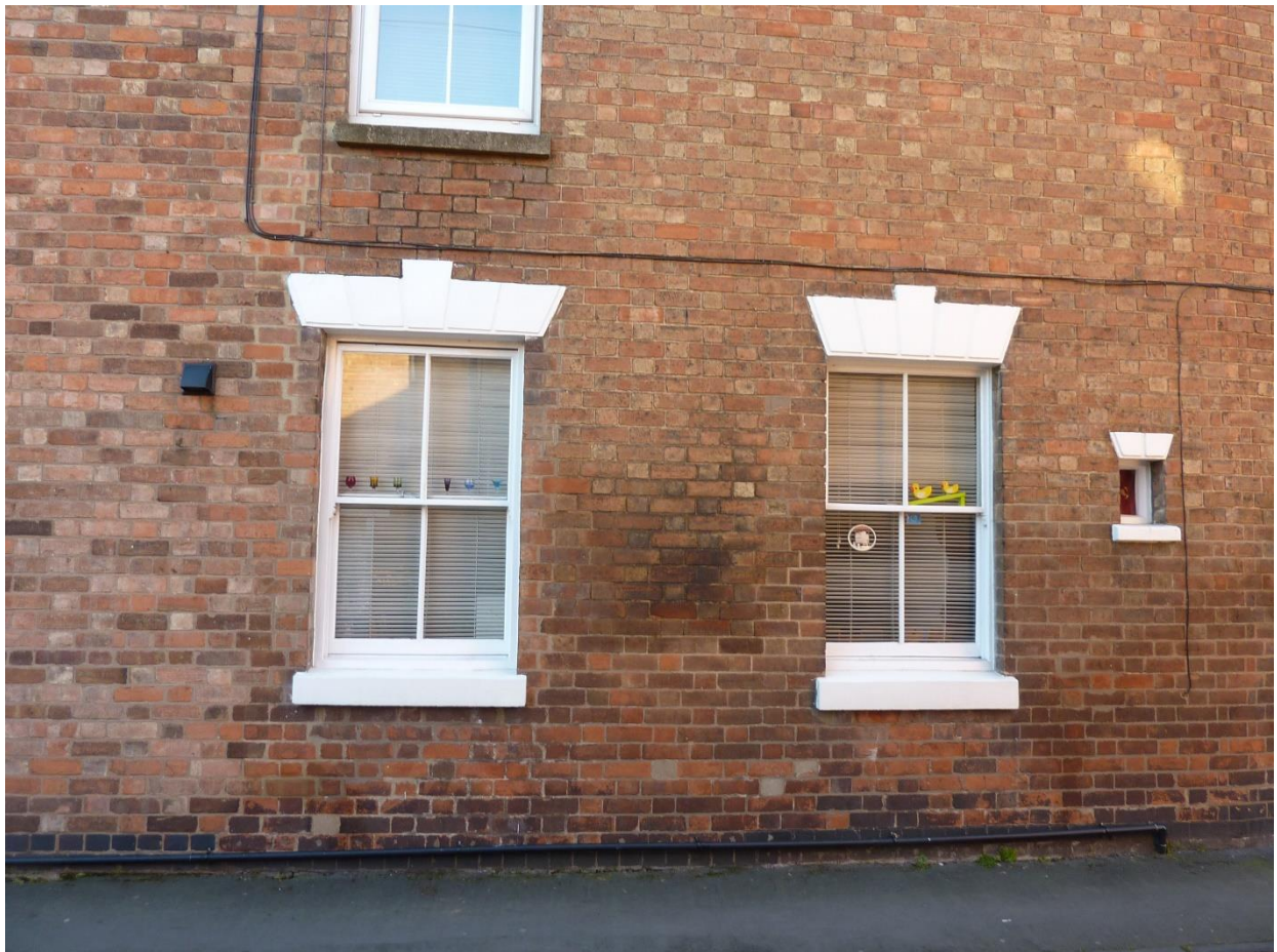
Fig. E12 - An example of windows with render used to create the effect of stone lintels. The windows have stone cills and sliding sash frames.
