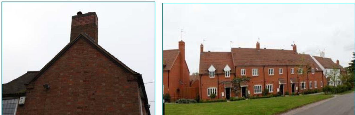
Fig. E19 - Examples of chimney in traditional and new dwellings.
