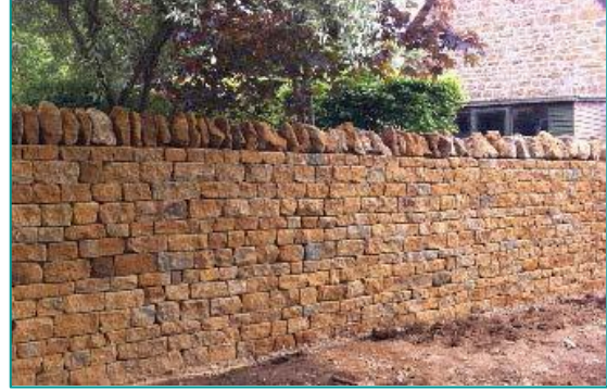
Fig. E5 - Hornton Stone wall (stone).
