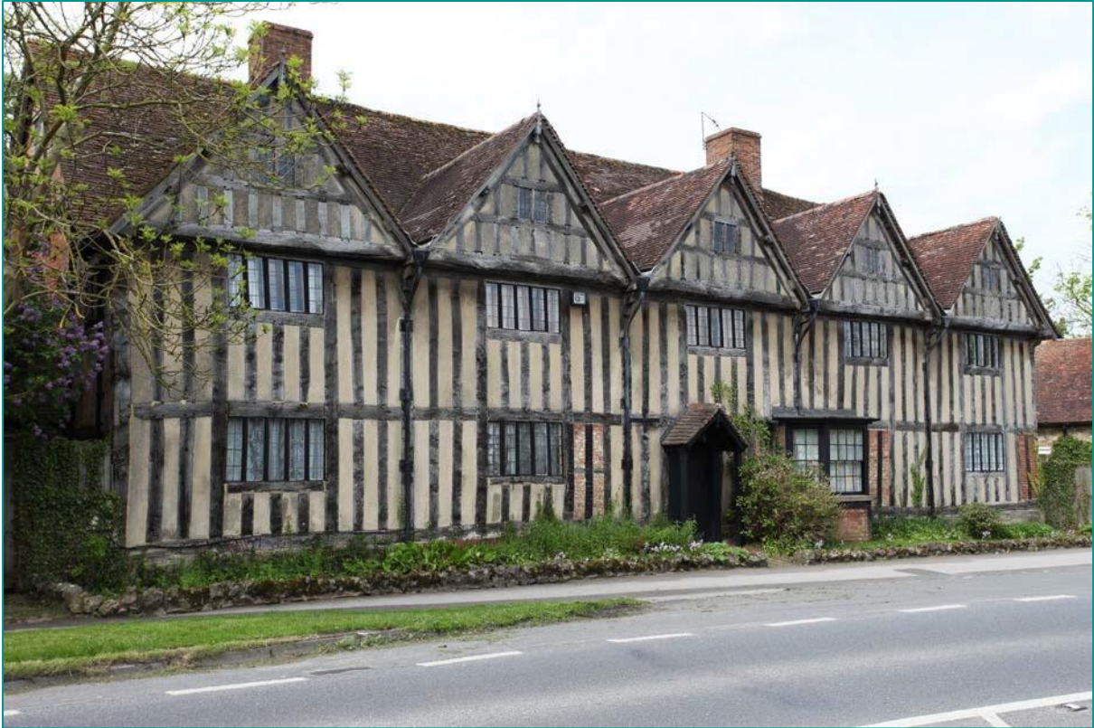
Fig. E1 - Photo of close studded timber framed house with rendered infill panels in Long Itchington, Feldon area.
