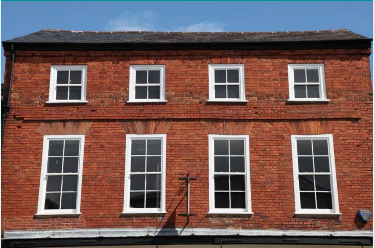
Fig. E 9 - Gauged brick flat arches on a house in Henley-in-Arden, Arden area. The openings are vertically aligned and the second floor windows are smaller than the first floor windows.
