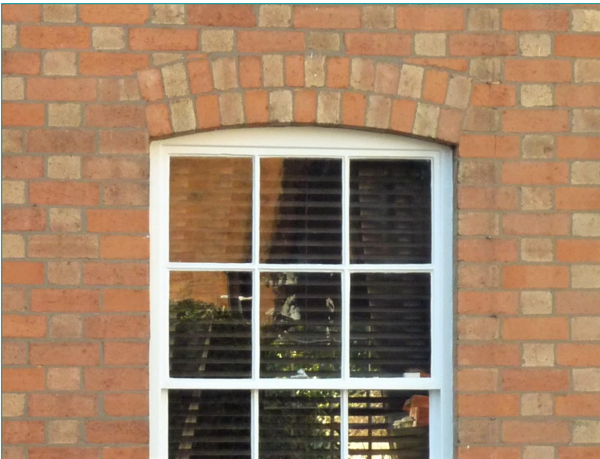
Fig E10 - Window with a segmental arch head. Note the arch is made up of headers on edge, a detail very characteristic of brick areas within the District.
