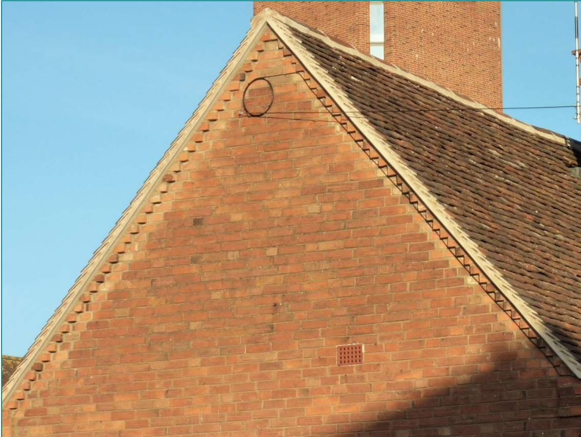
Fig. E17 – A trim verge of brick with stepped projecting header corbelling and a half-round ridge tile.
