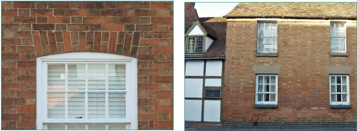
Fig. E2 - Photo of a brick house with rubbed brick flat arch window heads in Stratford on Avon.
