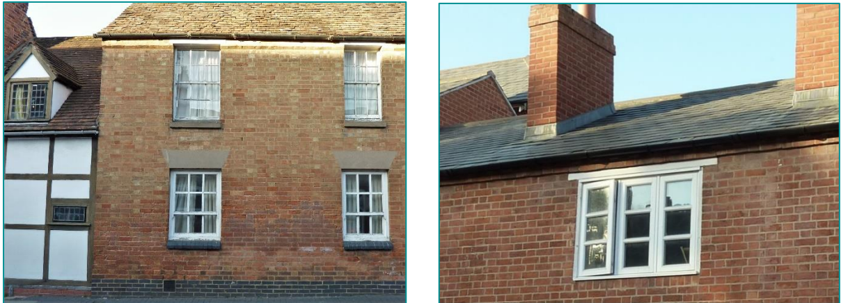
Fig. E11 - Cottages with windows set just below the top plate in Old Town, Stratford-upon-Avon. The casement windows shown are flush closing as opposed to 'storm proof'.
